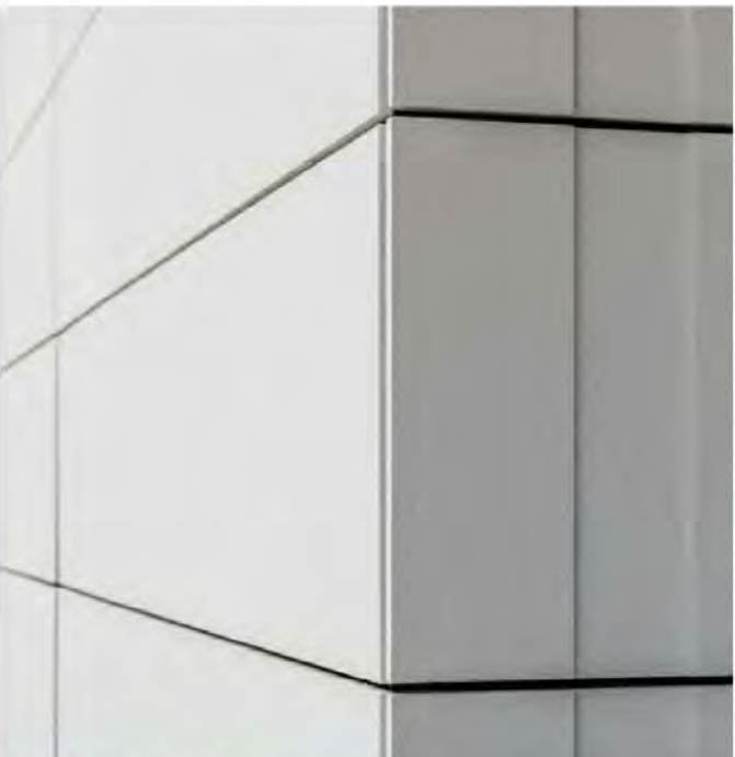
FRC PNL-1 Basis of Design: Taktl High Performance Concrete Panel Color: White, Texture: Smooth
