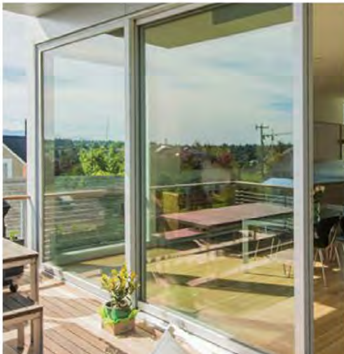
GL-1(T) Basis of Design: Solarban 72 Starphire Solar Control Color: Clear
